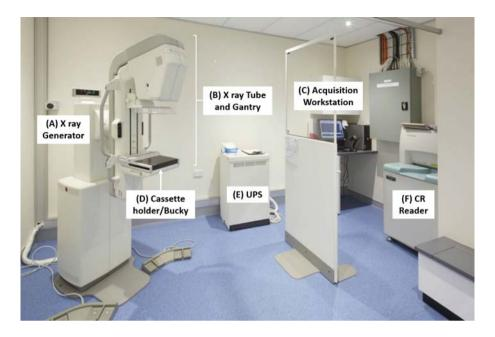
FIG. 16. Typical layout of a CRM equipment room. (Image courtesy of CPD Projects, Australia.)
